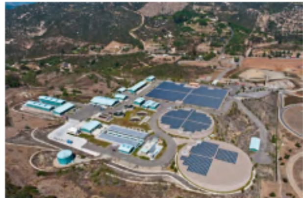
The 2003 Master Plan identified a need for additional water treatment for the region; the Twin Oaks Valley Water Treatment Plant was completed in 2008 (Water Authority, 2002).
