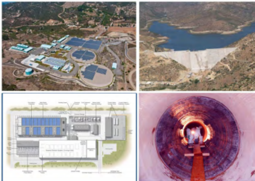
The 2003 Master Plan initiated and implemented many successful projects, including the Twin Oaks Valley WTP, the San Vicente Dam Raise, the Carlsbad Desalination Project, and various relining projects.
