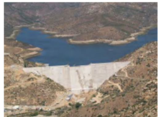
San Vicente Dam Raise. The San Vicente Reservoir expansion will provide regional storage for emergency conditions.
