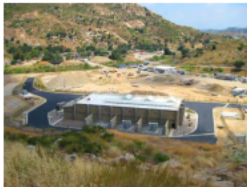
The San Vicente Pump Station will be utilized to supply untreated water during emergency events.
