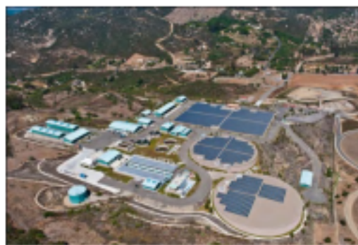
The Twin Oaks Valley WTP is a critical piece of infrastructure in the Water Authority's system, responsible for providing potable water deliveries to member agencies throughout the region.
